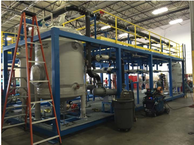
Pilot plant construction to be completed by 9/30/16
